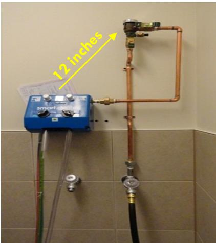
If an SVB is used, the backflow preventer must be installed 12" above the dispenser. If an RP is used, the backflow preventer can be installed below the chemical dispenser
